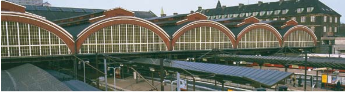
COPENHAGEN, CENTRAL STATION
